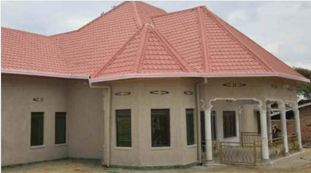
Private residence in Rwanda roofed with Versatile.
